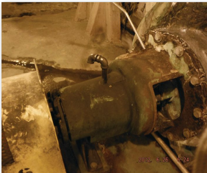
Figure 4: "Gooseneck" vents such as these should be avoided
